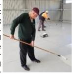
the last few weeks has been the painting of the entire shed floor with high grade two-pack epoxy coating. The coating will ensure easy cleanup of any
