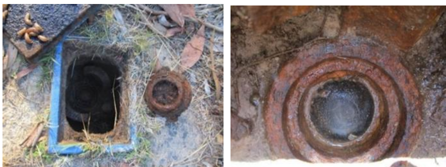
Figure 2: Example of FP Corrosion
