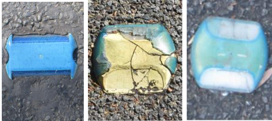
Figure 6: Example of Defective Road Markers
