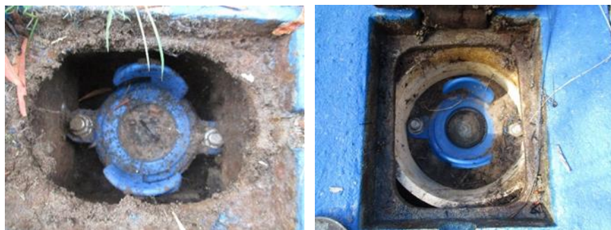
Figure 2: Example of FP Corrosion
