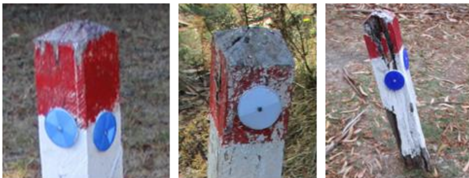
Figure 5: Worn or Flaking Red Paint on Marker Posts, Rotted Posts
